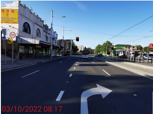
Streetscape along Anzac Parade to the south
