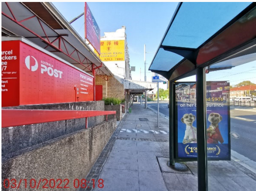
Footpath along Anzac Parade to the south
